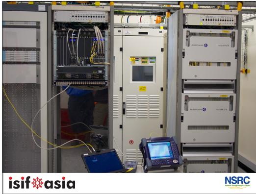
Tonga-Suva Landing Station: The Alcatel-Lucent 1620 Light Manager (LM) SLTE (Submarine Lightwave Transmission Equipment) is a DWDM terminal for use in repeatered submarine cable systems. It can be used on systems operating at  $N \times 10 \text{ Gb/s}$ , either as an upgrade for existing systems, or as a terminal for new systems. It supports up to  $192 \times 10 \text{ Gbit/s}$  channels, with system capacity
